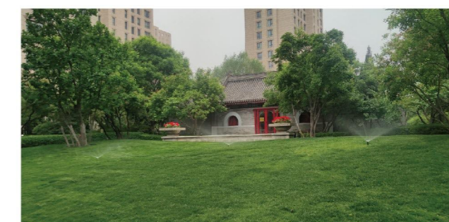
Sprinkler irrigation system of Wangjing Jinmao Residence raises the utilization level of water for greening
