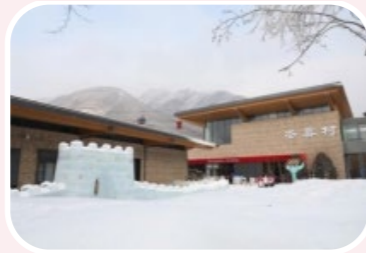
金隅砂漿助力延慶冬奧村建設 BBMG's mortar in the construction of the Winter Olympic Village in Yanqing
