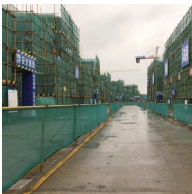
腳手架覆網 Scaffold Coverings
