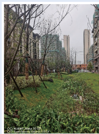
散水草溝 Scattered water grass ditch
