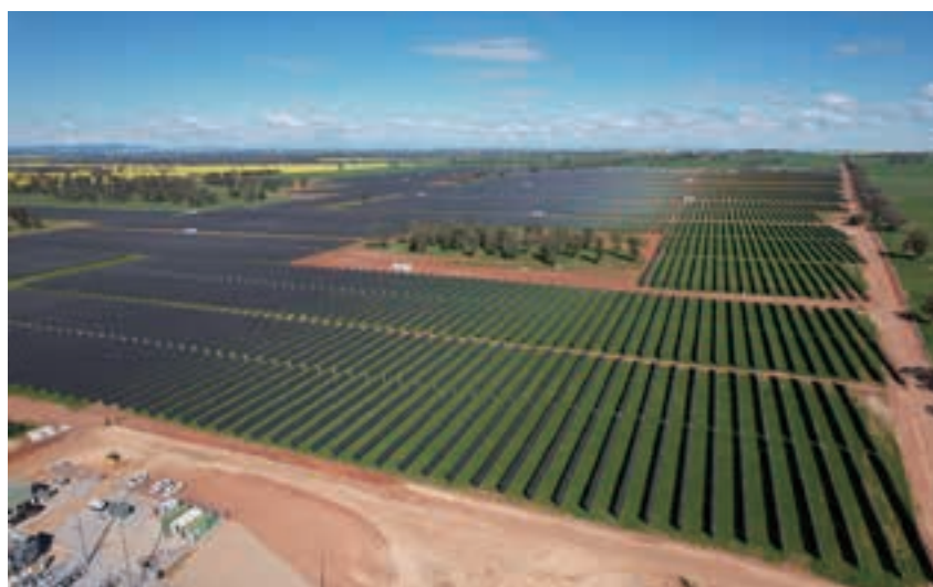
Victoria Power Networks 太陽能裝置
