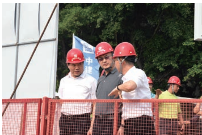
▲ Group leaders inspect construction in progress
