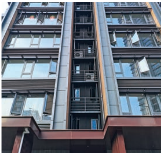
▲ LOW-E transparent hollow tempered glass
