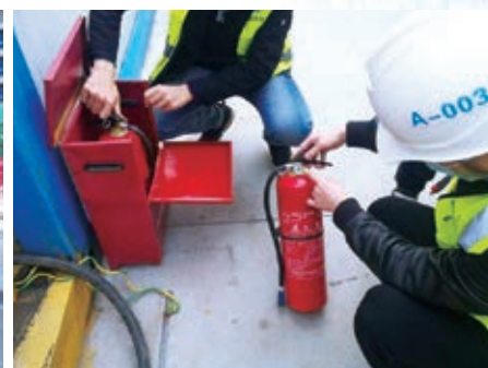
▲ Fire safety inspection of construction in progress
