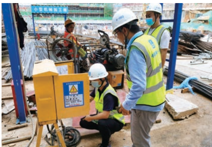
▲ Third-party safety inspection
