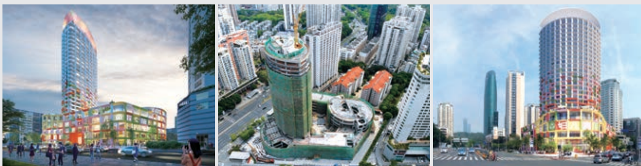
▲ Shenzhen Women and Children Tower Renovation PPP Project
