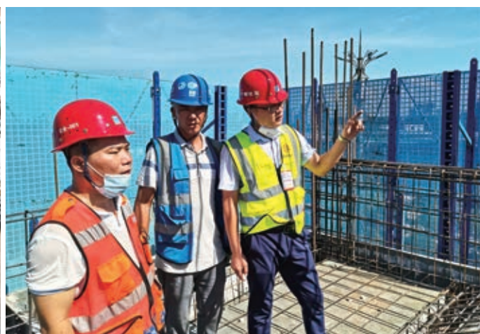
▲ Third-party safety inspection
