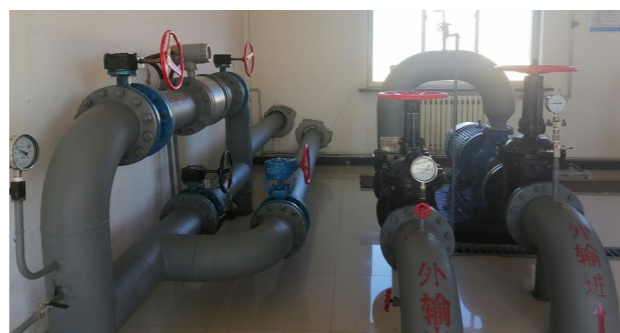
Renovation of the sewage transportation system in Yuedong oilfield
