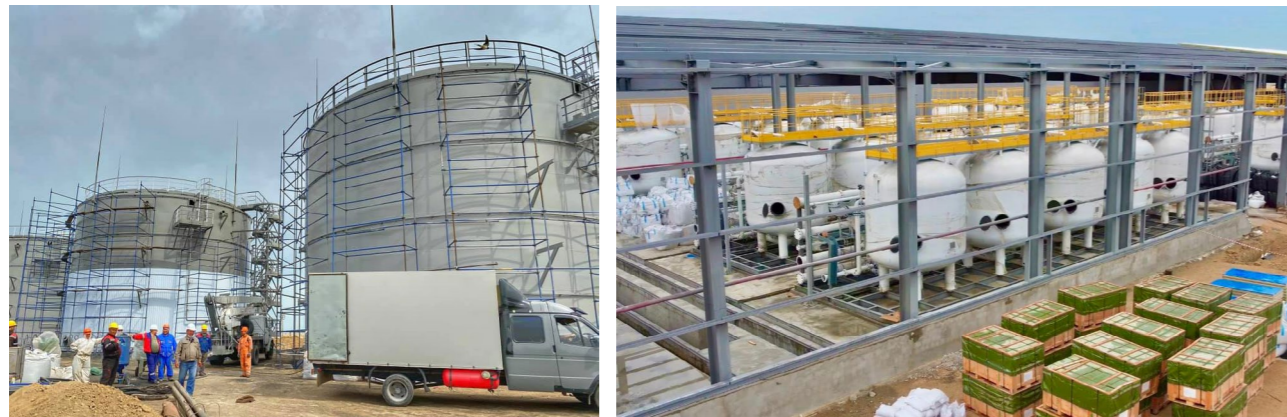
Sewage treatment plant under construction at Karazhanbas oilfield
