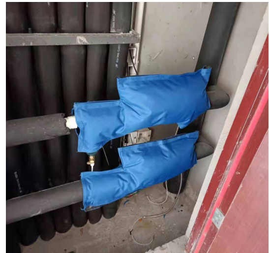
Installing electric heating sleeve for water pipes
