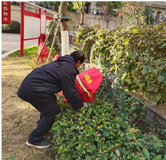
Installing heating sleeves for fire hydrants
