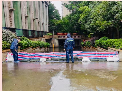
On-site flood prevention
