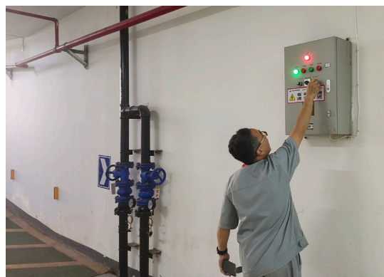
Inspection on basement sewage pump
