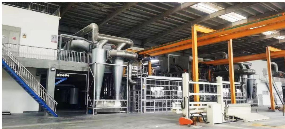
Production workshop of a company
