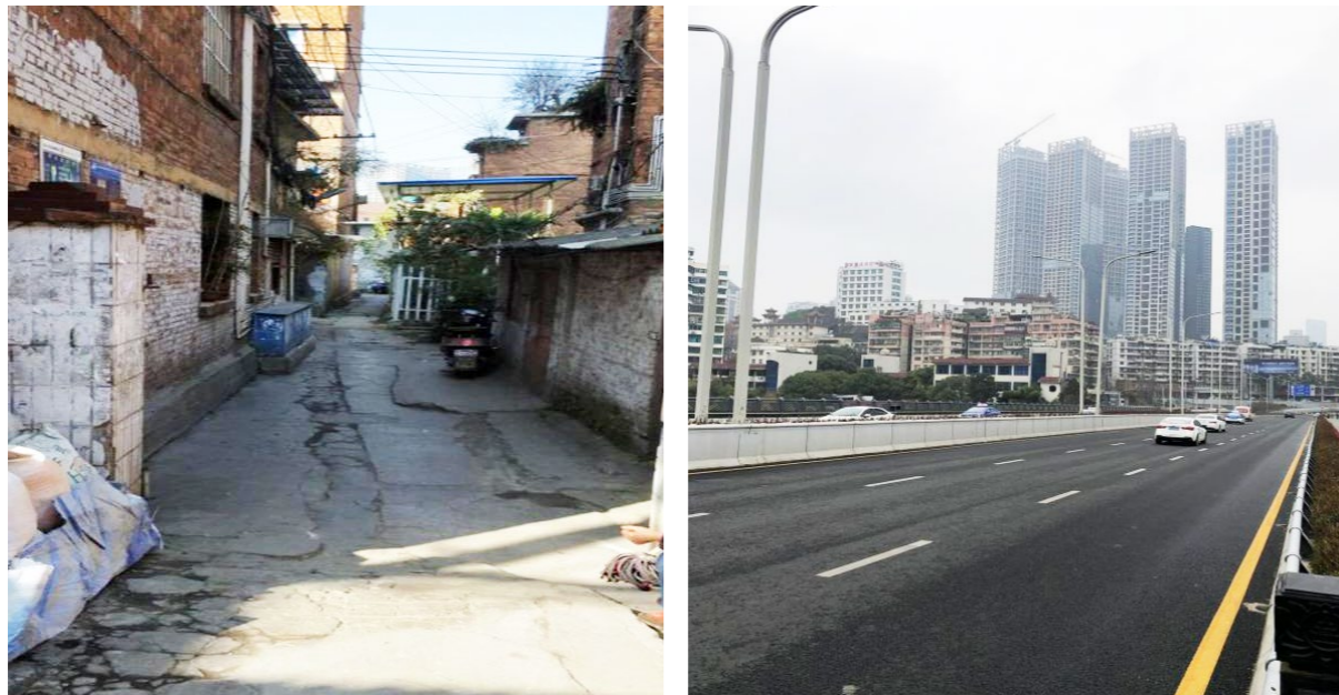
Before and After of the "People's Avenue" urban construction project in Guiyang
