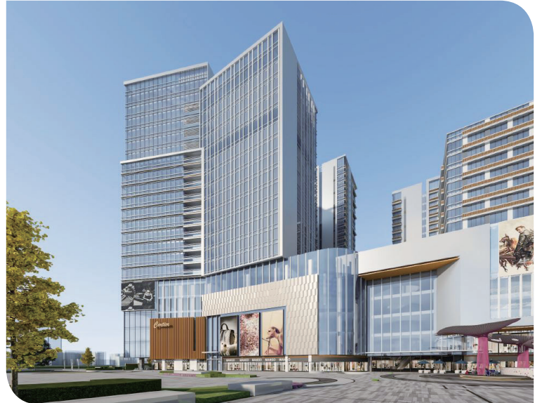
Commercial/office towers of Regal Cosmopolitan City (*)
