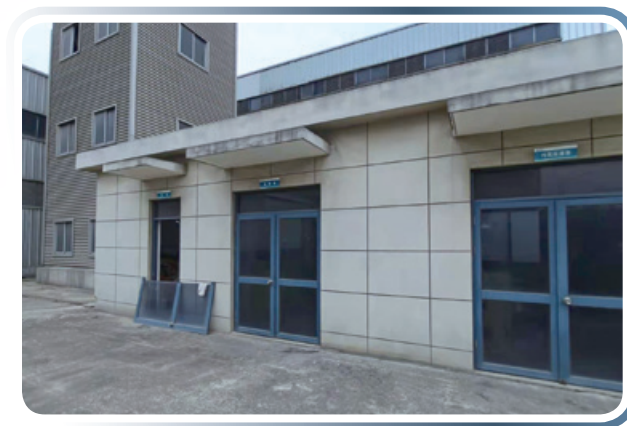
Sewage treatment facilities at Taizhou factory 台州工廠污水處理設施
