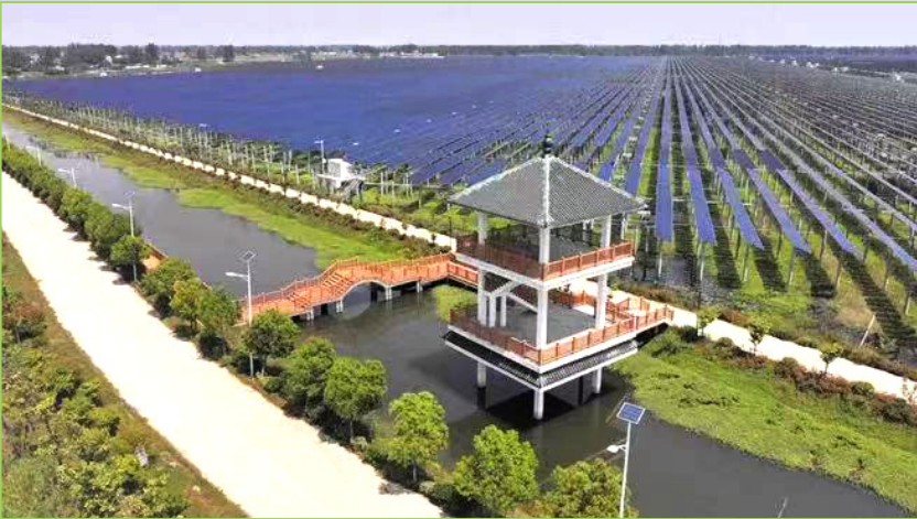
Shouxian Solar Farm
