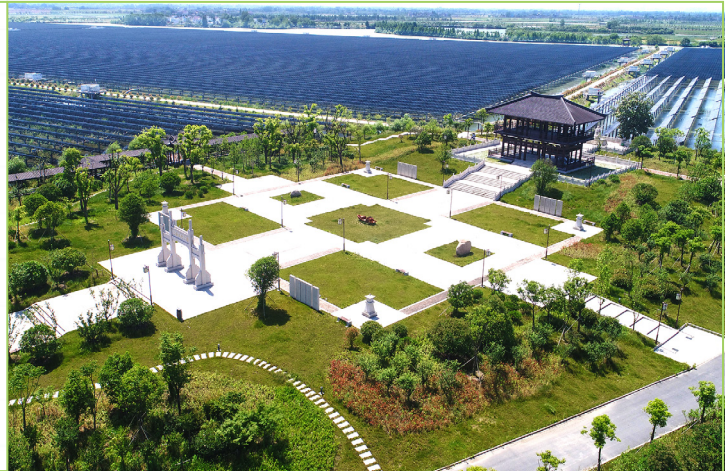
Fanchang Solar Farm
