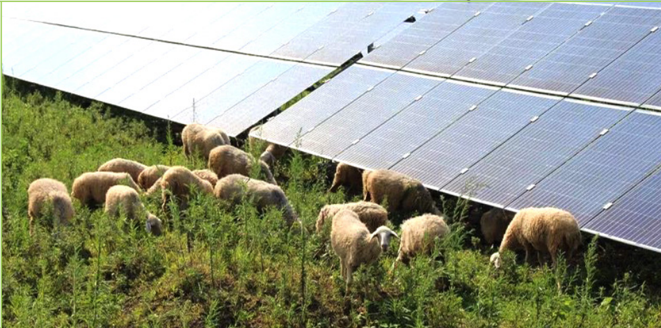
Jinzhai Solar Farm
