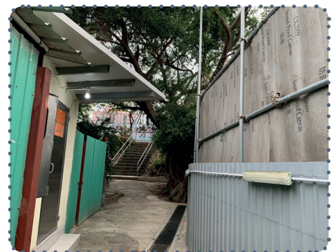
Noise barriers on-site
