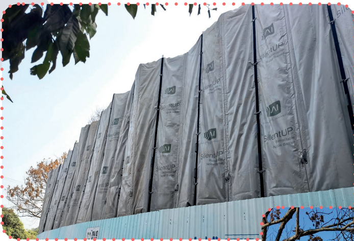
Noise barriers on-site
