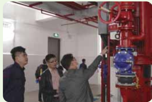
項目設備房參觀 Visits to project equipment room
