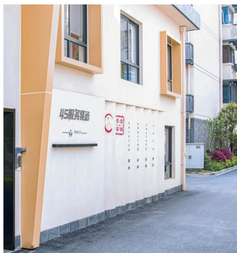
“4S Service Station”
