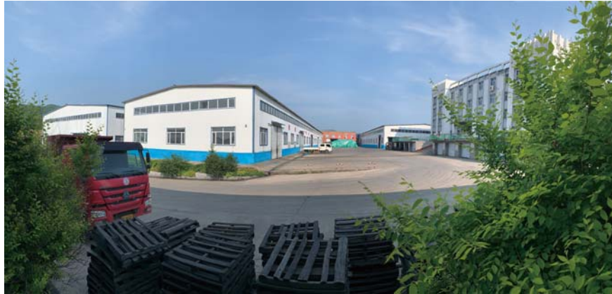
Figure 8–8: Spherical graphite processing plant
