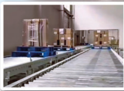
連廊智能運輸系統 Intelligent Transportation Systems
