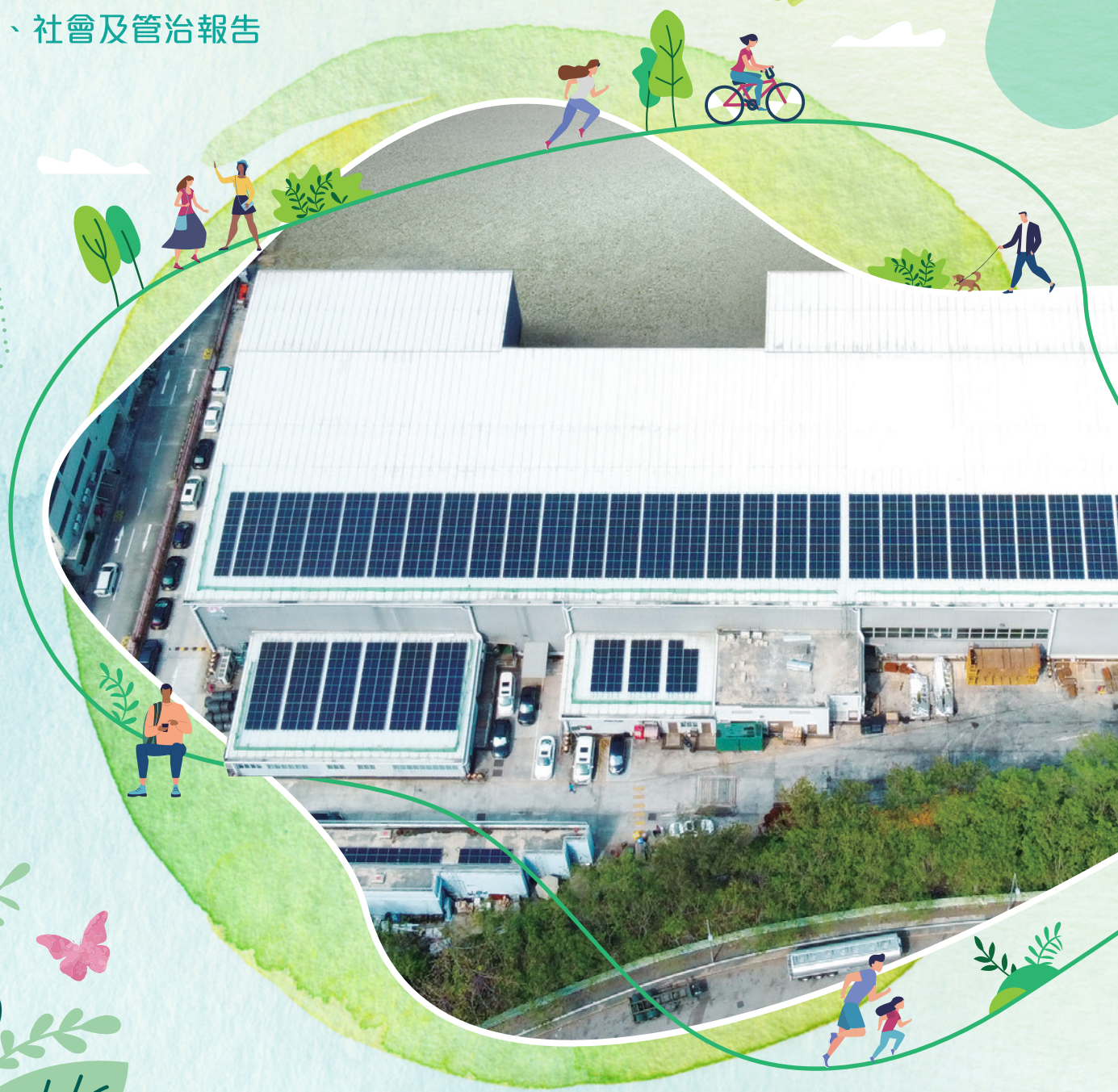
Automated Rebar Processing and Assembly Plant in Tsing Yi 位於青衣的自動化鋼筋加工及裝配廠
