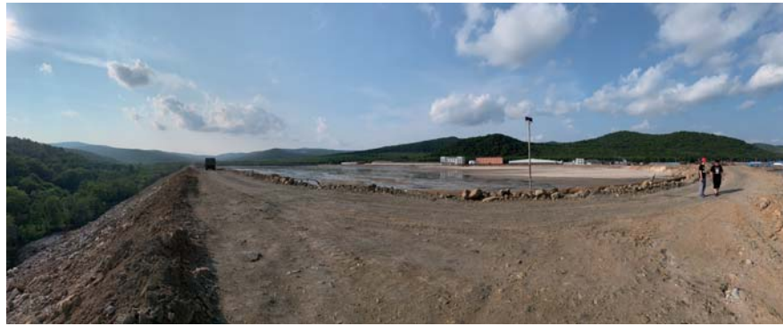
Figure 8–7: Current tailings storage facility, looking from the southeast to northwest
