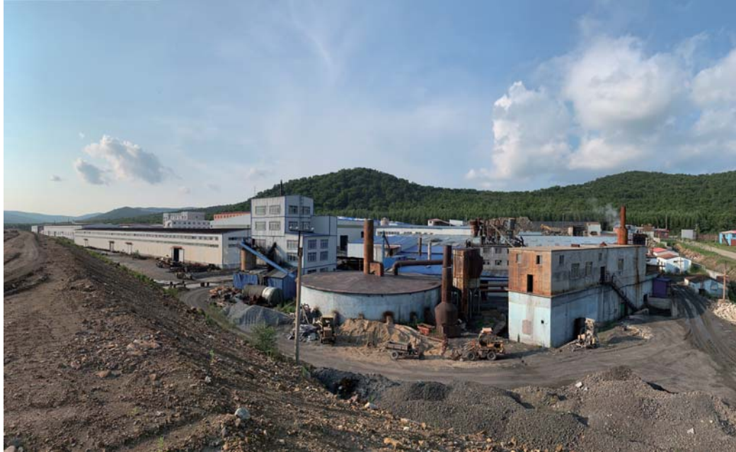
Figure 8–4: Panoramic view of China Graphite’s beneficiation plant, tailings storage facility and spherical graphite processing facility
