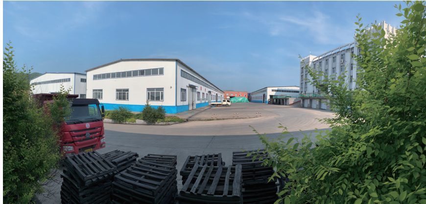
Figure 8–8: Spherical graphite processing plant
