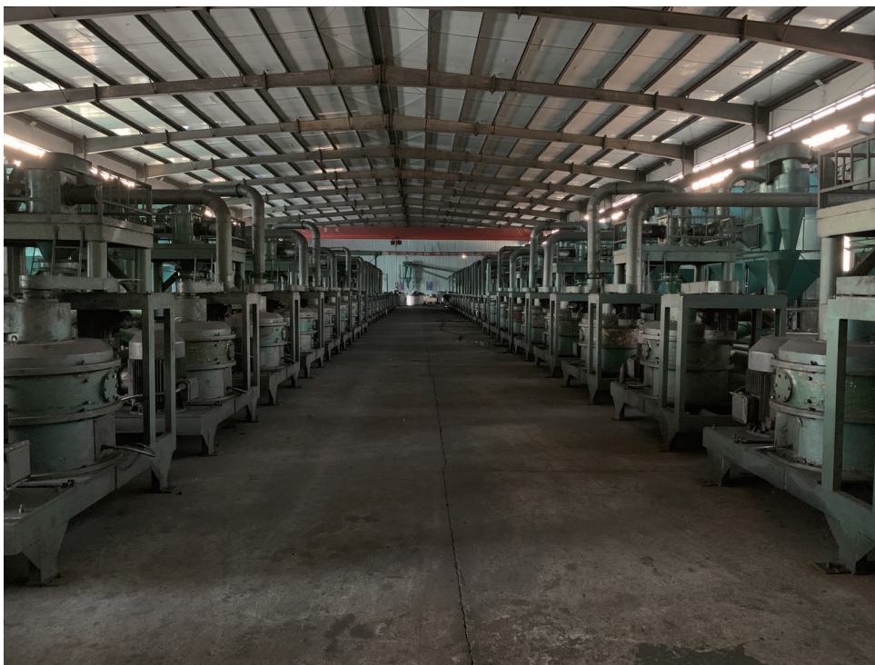
Figure 8–9: Rounding circuit in the spherical graphite processing plant
