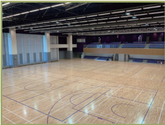
Design, supply and installation of hardwood sport flooring system for sports centre in Area 1, Tai Po 大埔第1區之體育館－設計、供應及安裝運動木地板系統
