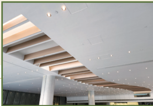
Design, supply and installation of cement board ceiling system at balcony and G/F of The Hong Kong Palace Museum for The West Kowloon Cultural District Authority 西九文化區管理局香港故宮文化博物館－設計、供應及安裝露台及地面層之水泥板天花系統
