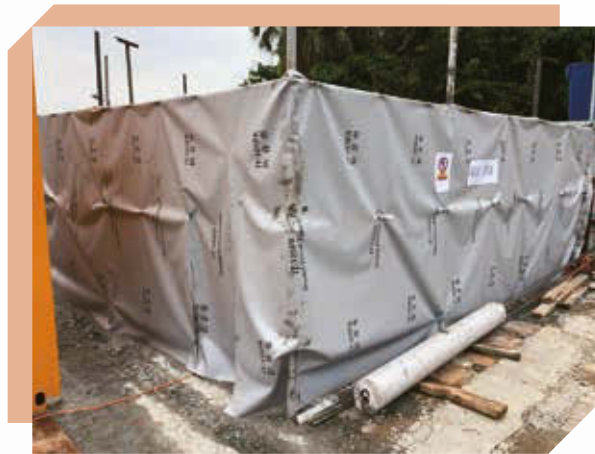
▲ Noise Barrier enclosed the workplace 工地周圍設有隔音屏障
