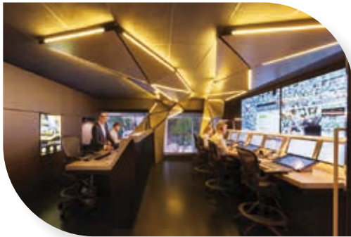
Central monitoring system, Care Assist
