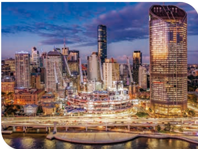
Construction at Queen's Wharf, Brisbane
