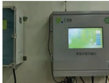
Sewage pollutant monitoring devices installed at the Zhongshan factory
