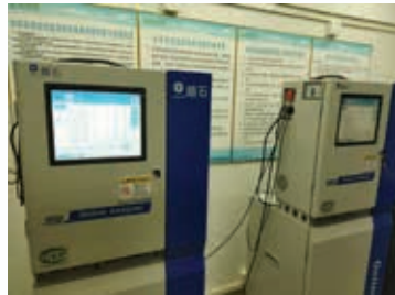
Sewage pollutant monitoring devices installed at the Zhongshan factory
