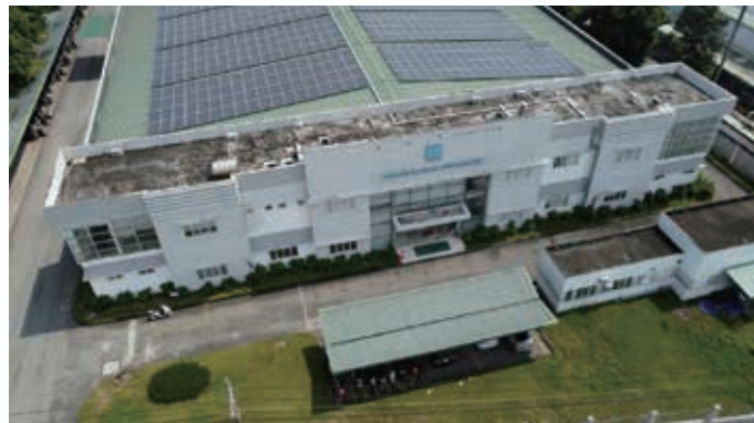
Solar PV System in Vietnam Factory
