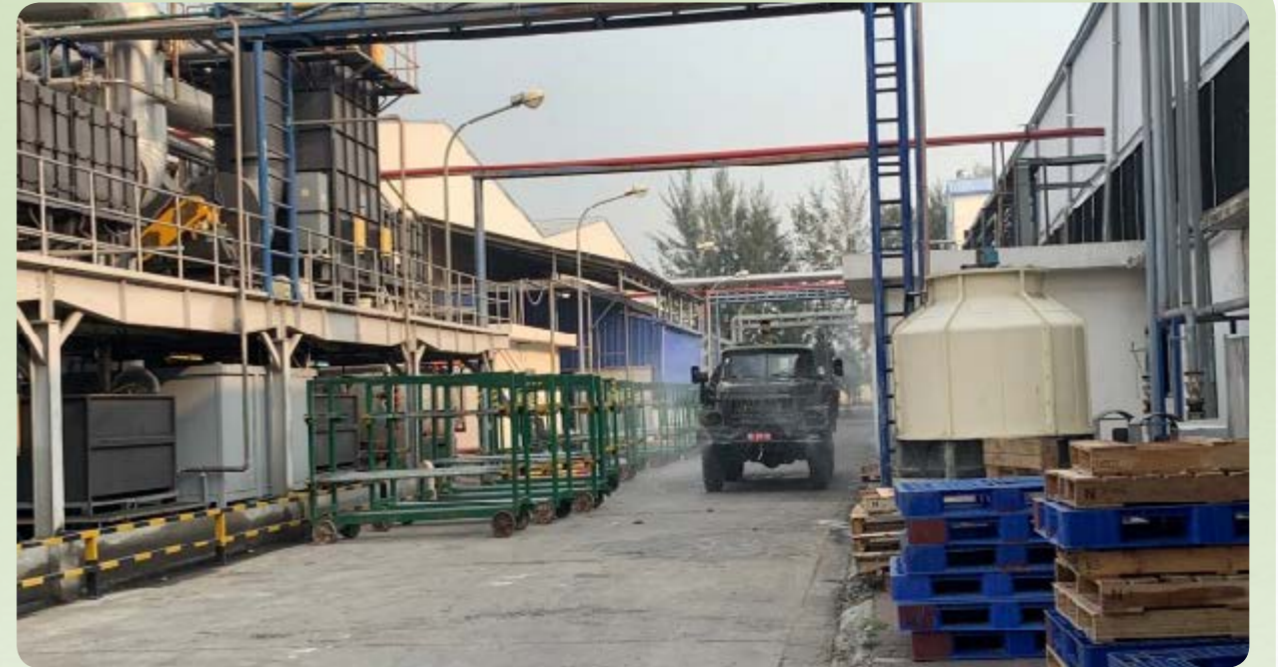
Disinfection Work for the Plant - Vietnam Plant
