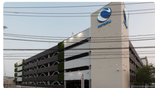
NIRAKU Ebina Hongo hall's multi-story parking lot
