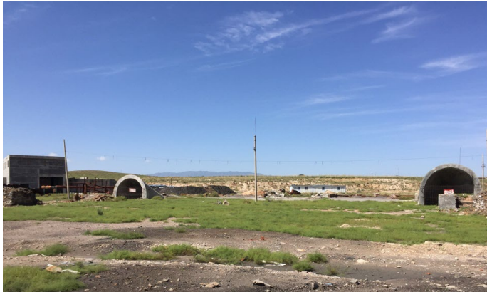
Figure 23: Yong-an Surface Plant Area – View of Two Inclined Shafts and Ventilation Fan Structure in the Background
