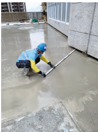
Floor screeding works
