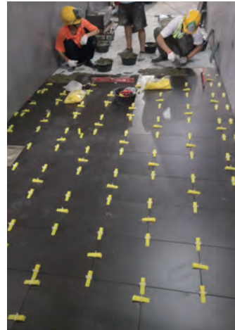
Tile laying works
