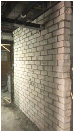
Brick laying works
