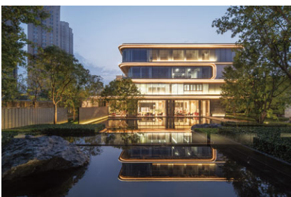
天津鉅悅公墅 Tianjin CIFI Park Mansion
