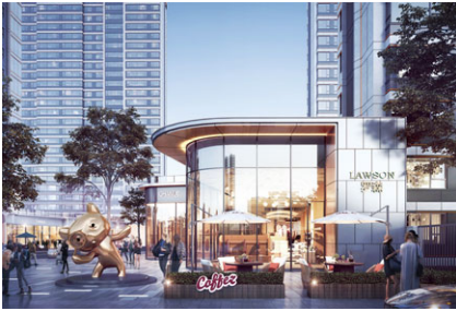
南京江北晴翠府 Nanjing Jiangbei Qingcui Mansion
