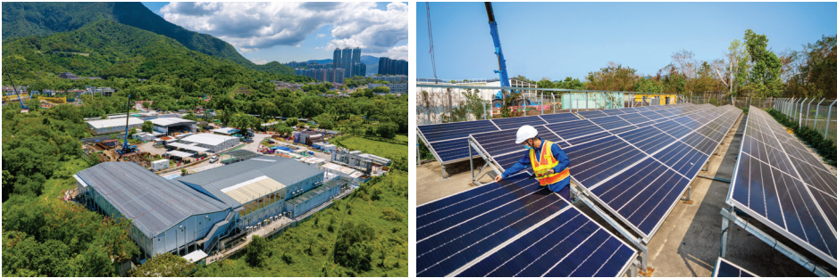
Solar panels in construction site in Shap Sze Heung
