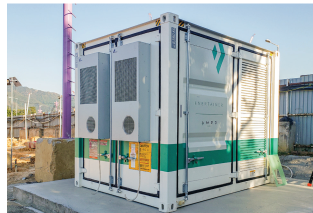
Enerainers at construction sites
