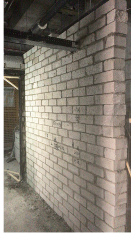
Brick laying works
