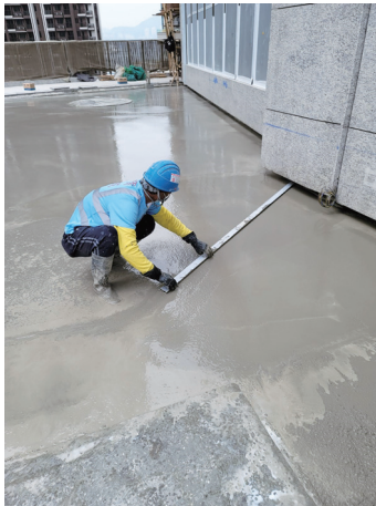
Floor screeding works
