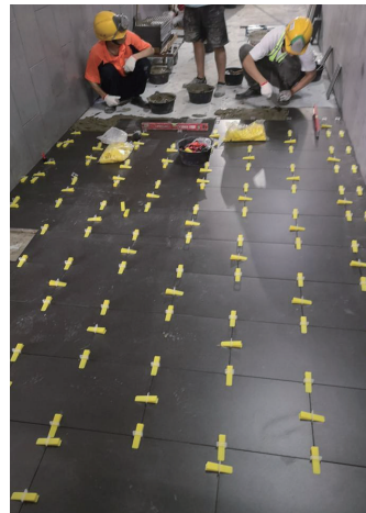
Tile laying works
