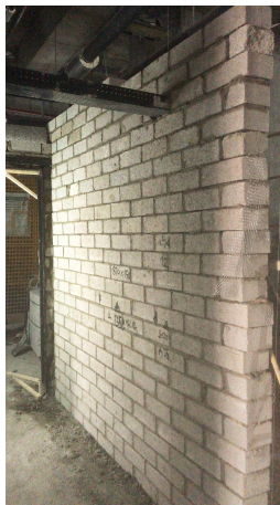
Brick laying works
