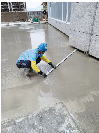
Floor screeding works
