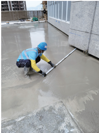
Floor screeding works
