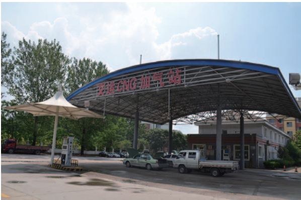
No. 2 Refuelling Station
