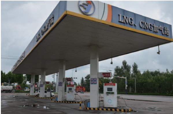
Longtan Road LNG and CNG Refuelling Station
