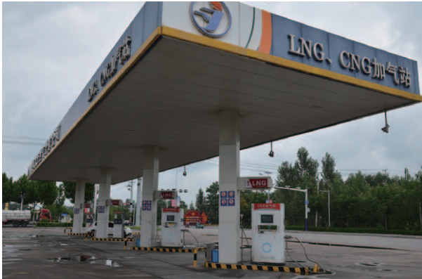
Longtan Road LNG and CNG Refuelling Station
