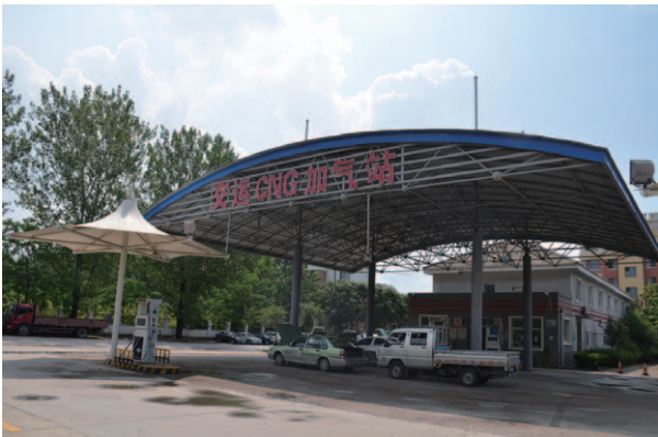
No. 2 Refuelling Station
