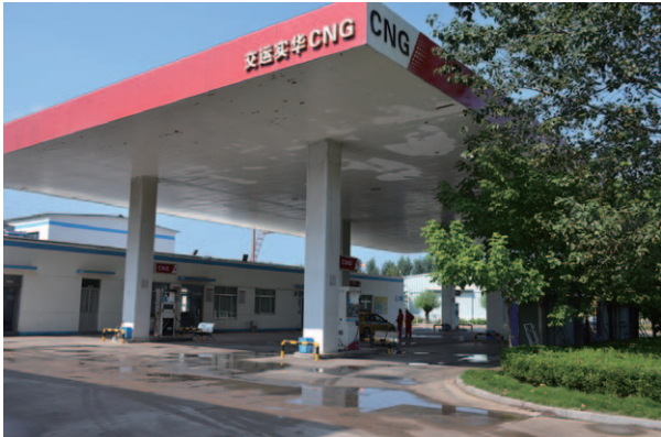
No. 1 Refuelling Station
