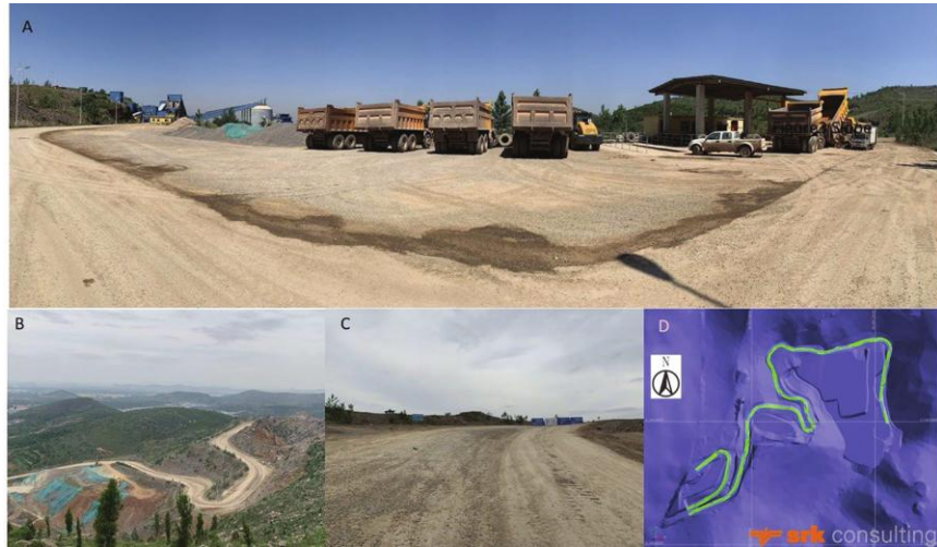
Figure 6-2: Quarry current conditions
