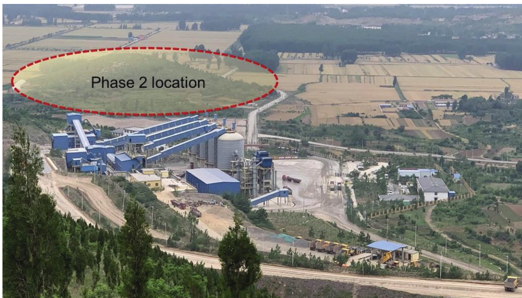
Figure 8-1: Existing and proposed approximate location of the Phase II processing plant, looking west
