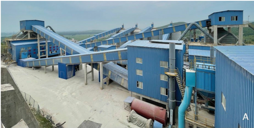
Figure 8-4: Phase I processing plant
