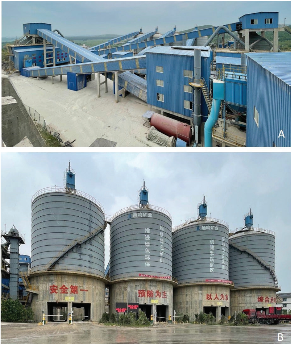
Figure 8-4: Phase I processing plant
