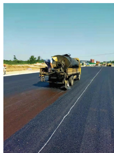
Asphalt concrete (emulsified)
