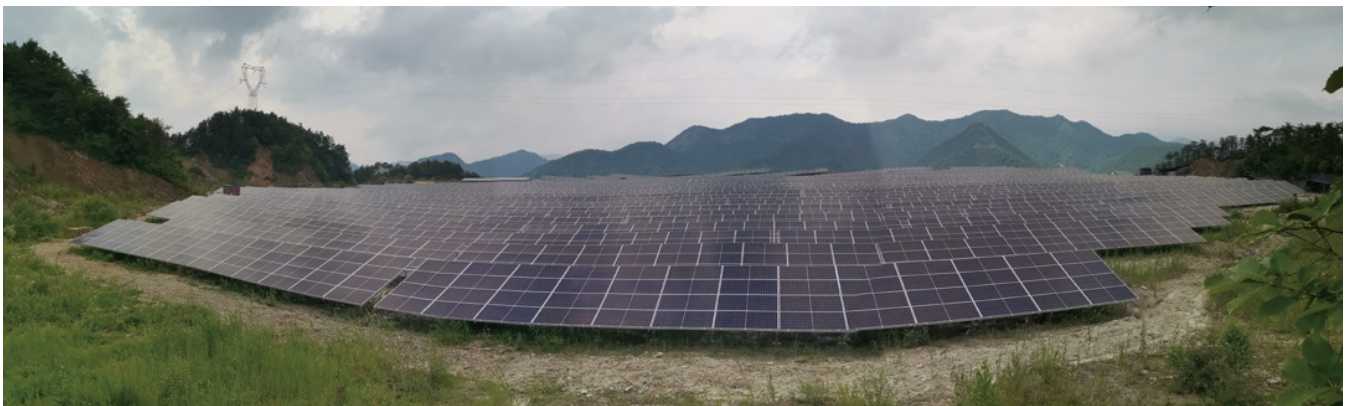
■ The Liushuigou TSF solar power generation project installed 9,000 solar panels on a closed tailing pond, with an installed capacity of 12 MW. The project will gradually be connected to the grid and is expected to generate 19.87 million kWh of electricity each year.
