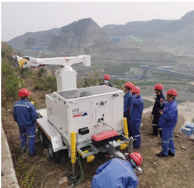
At our Chinese operations, we installed the IBIS ArcSAR radar system to complement our existing slope surveillance system and improve our slope safety and alert mechanisms.
