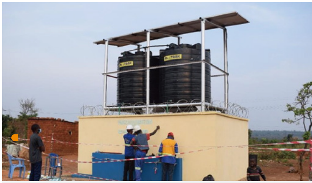
■ KFM installed a solar-powered water pump for members of the local community. In addition to promoting the use of clean energy, the new pump has reduced the financial burden on local residents by lowering energy bills.
