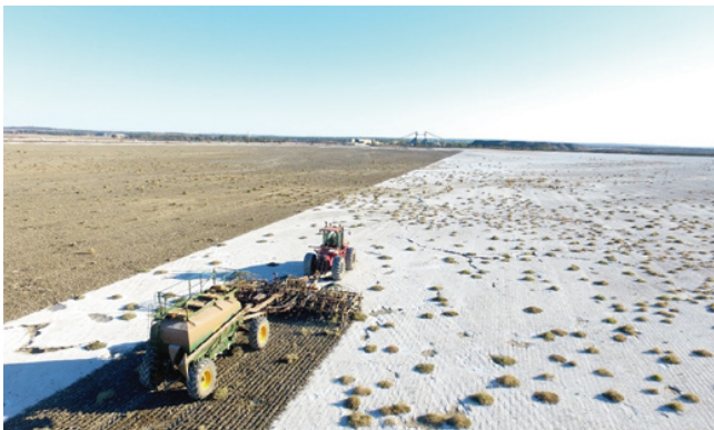
Our NPM mine in Australia successfully established a barley crop on a tailings storage facility. This offers a low-cost, simple, and effective way to suppress dust.
