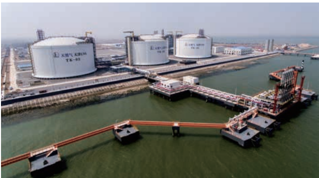
Sinopec Tianjin liquefied natural gas (LNG) project
