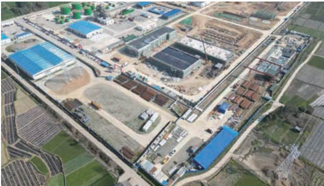
The desulfurisation station project of Leikoupo Formation Project in West Sichuan Gas Field
