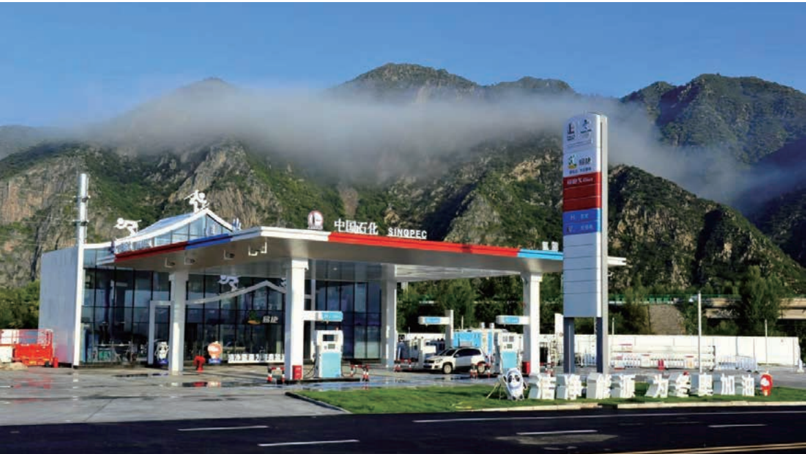
Sinopec Engineering Incorporation built Xiwanzi Winter Olympics Hydrogen Fuelling Station
