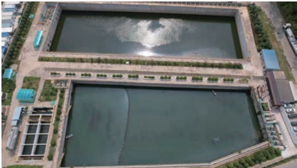
Sedimentation tanks were built to reduce wastewater discharge
