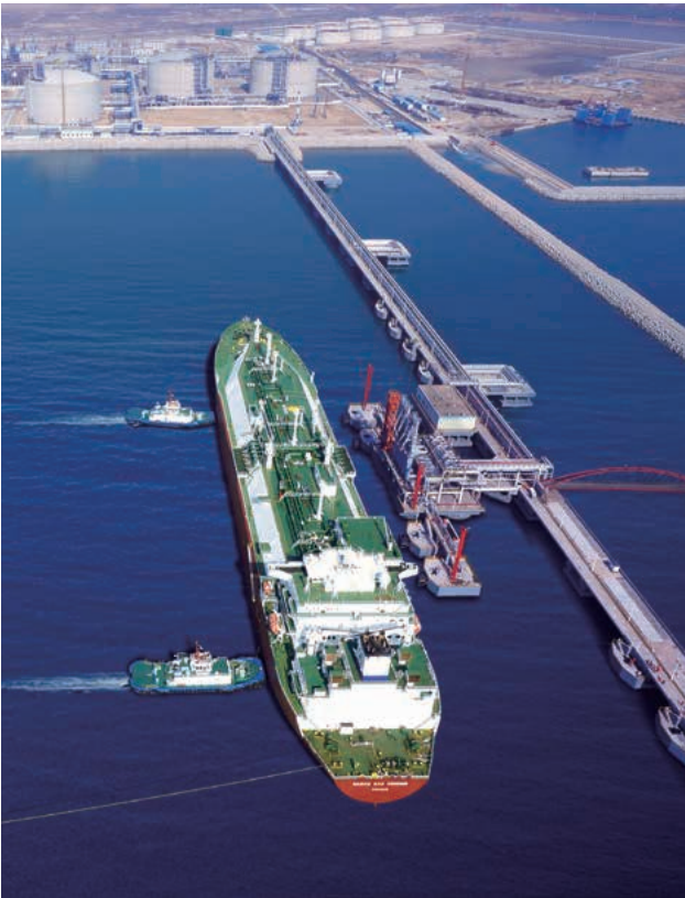
Sinopec Shandong liquefied natural gas (LNG) project
