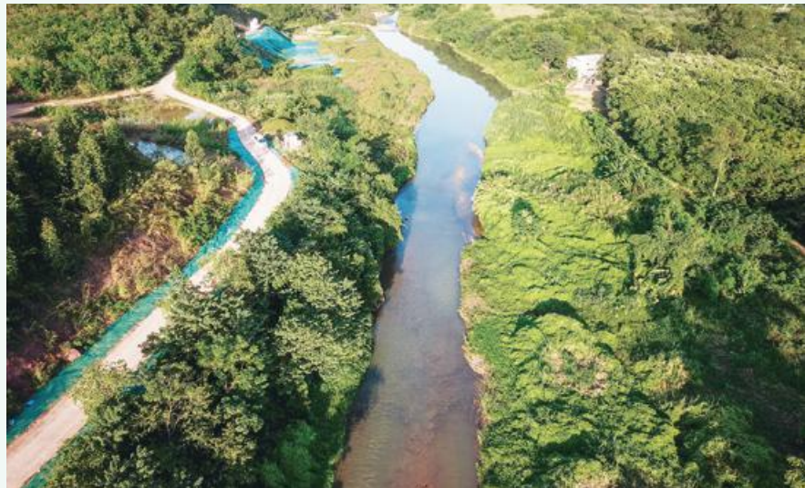
Nanning Shuitang River Integrated Restoration PPP Project 南寧水塘江綜合整治工程PPP項目
