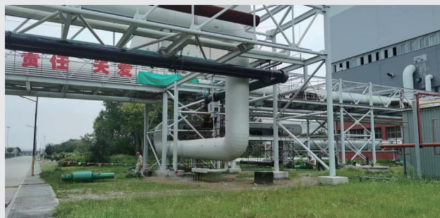
Pipe Network of Units for Increasing Capacity to Supply Industrial Steam
