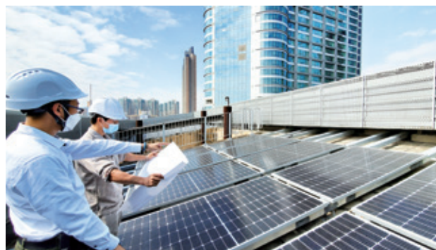
Additional solar panels were installed at both properties in 2022 to leverage sunlight for more renewable energy.
