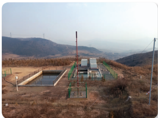
Figure: Skid-Mounted Sewage Treatment Unit of Panzhuang Project
