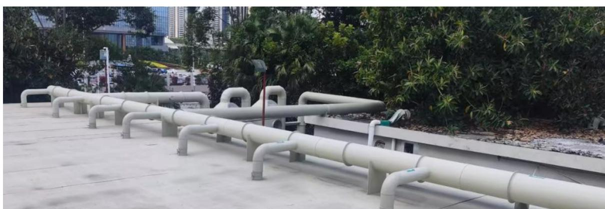
The pool of the wastewater station is capped to reduce gas escape
