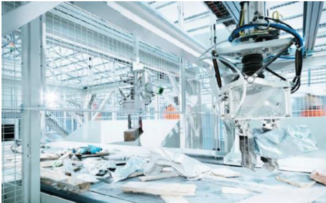
Photo: Suzhou Branch supported the construction of Kunshan Bulky Waste Crushing Center, where the crushed scraps could be recycled through advanced technologies
