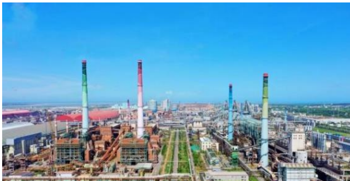
Photo: CCB facilitating the launch of the Baowu Green Carbon Fund. In the photo is the industrial heritage conservation and reuse project at China Baowu Steel Conference and Exhibition Center
