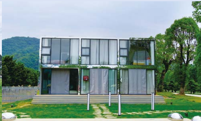
Picture 16: Building on flat ground (after erection)
