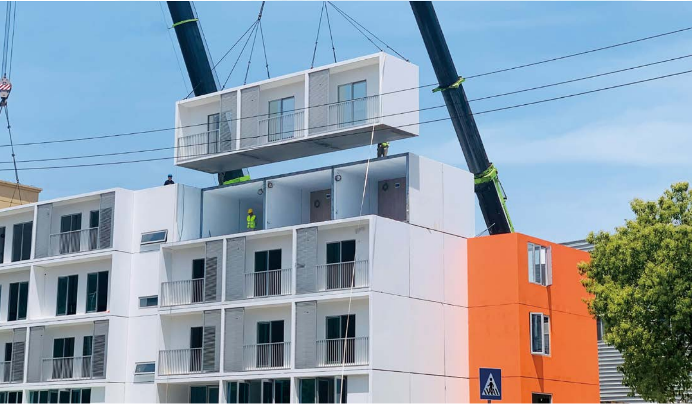
Picture 11: Real shot of the installation of Broad Homes Mofang's apartments
