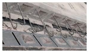
Picture 2: Shear key replacement for rough surface process
