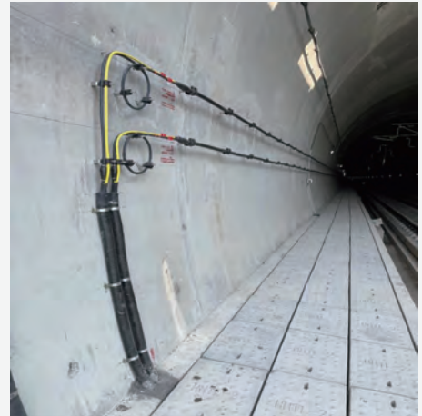
▲ Hangzhou-Huzhou Railway public network coverage project
