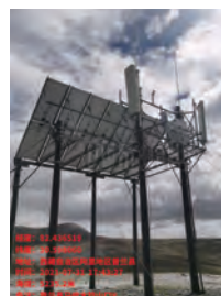
▲ Solar photovoltaic power supply for base station
