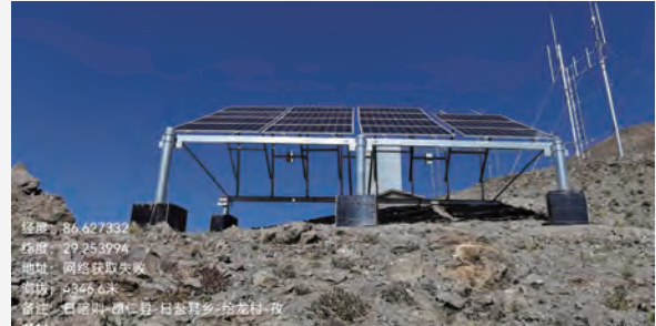
▲ Construction of solar base stations in Tibet
