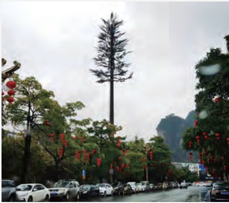
▲ Bionic tree base station in Bama Changshou Village coexists harmoniously with the surrounding environment
