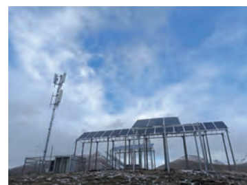
▲ Solar photovoltaic power supply for base station
